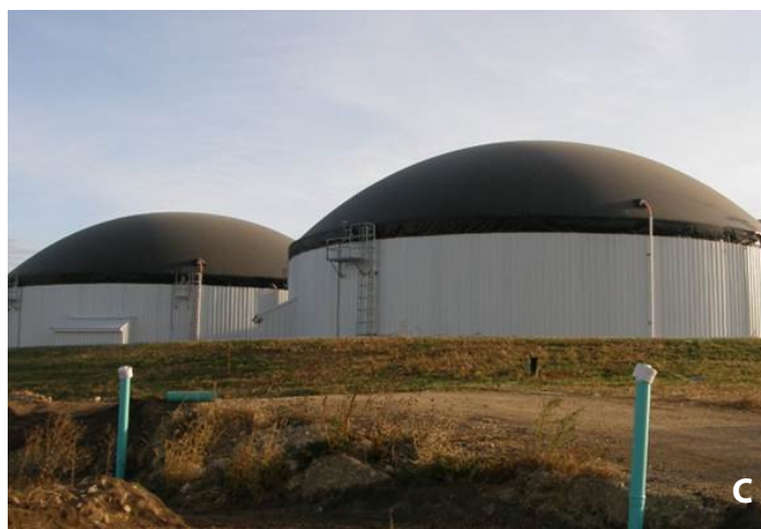
Figure 3. Types of anaerobic digesters: a) Covered lagoon, b) plug-flow, and c) complete mixed.
