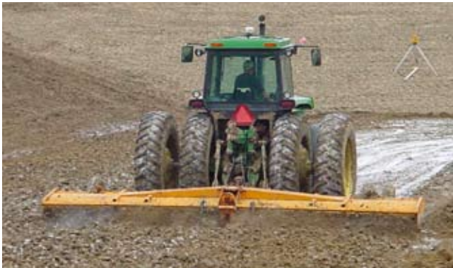
Figure 10D-23 High-speed rotary mixer used to mix dispersants into clays ( Photo credit Jody Kraenzel, NRCS )
