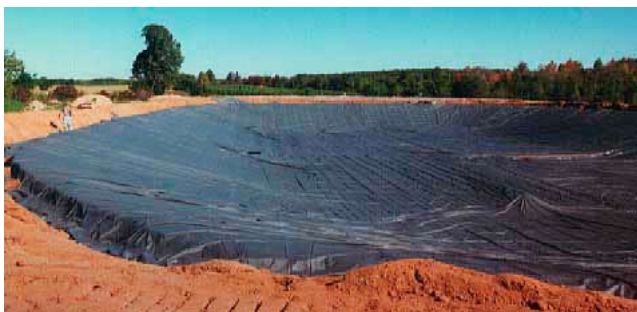
Figure 10D–6 Agricultural waste storage impoundment lined with a geomembrane ( Photo credit NRCS )
