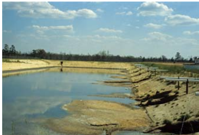
Figure 10D–1 Animal waste storage pond constructed before the implementation of modern design guidelines
