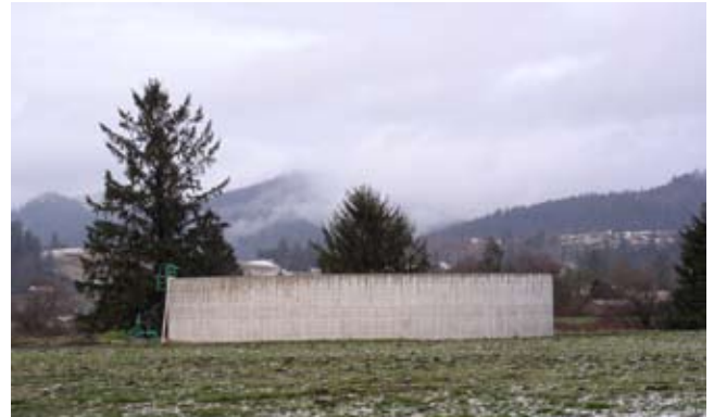
Figure 10D-4 Aboveground storage tank for animal waste ( Photo credit Mitch Cummings, Oregon NRCS )
